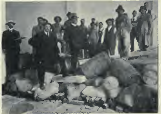
Fig. 2—Concrete test. Curry Building, Winnipeg, Man.
